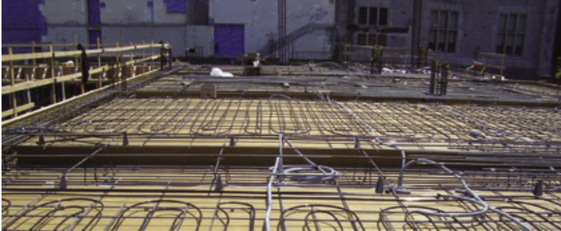
Earth Tech's award-winning system for the Learning Centre.
